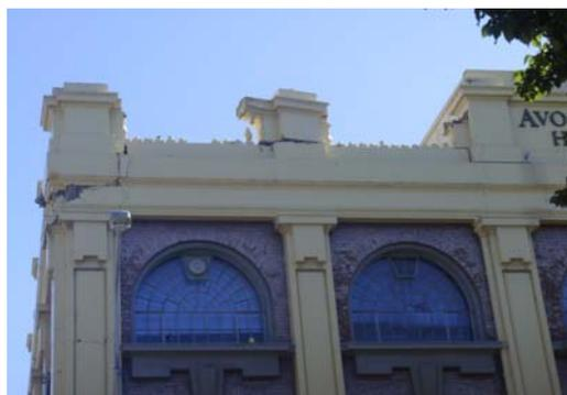
Figure 1. Damage to Avonmore House in the 2011 Canterbury Earthquake.
